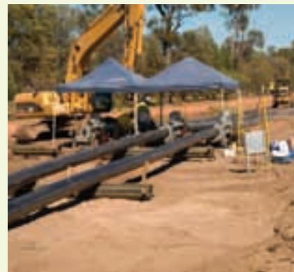
Butt welding the twin gas and water pipelines prior to installation
