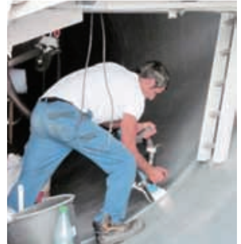
Extrusion welding the inside of the spigot – socket joints
