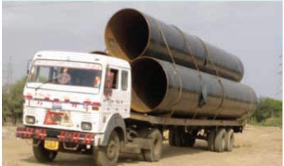
Some of the large diameter coated steel pipes being transported to site
