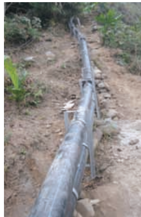
200mm rising main pipeline erected with mechanical clamping
